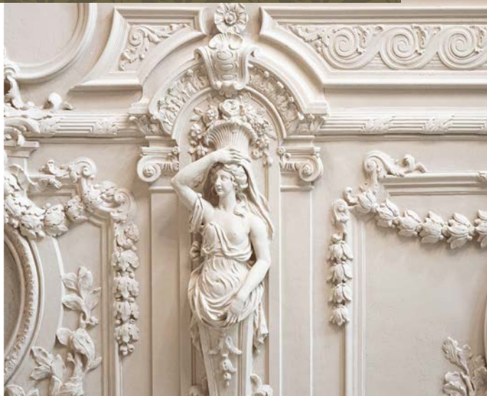
Rosecliff Ballroom ceiling detail
