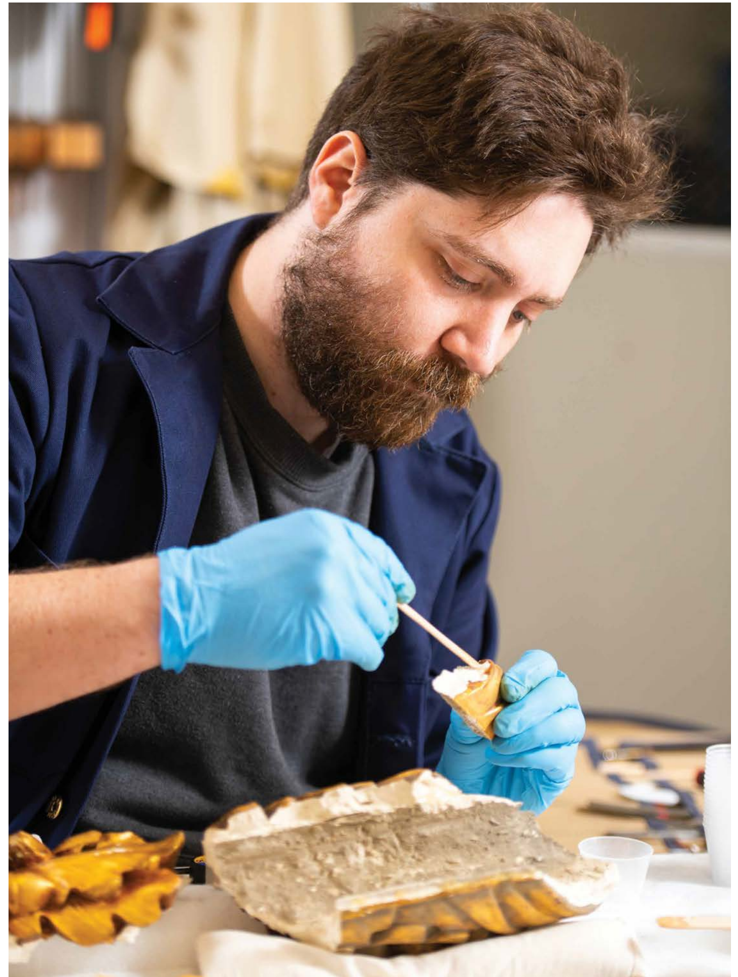
Collections Care Specialist Dogan Farancz repairs gilt decorative plaster elements from the Gold Room ceiling at Marble House.
