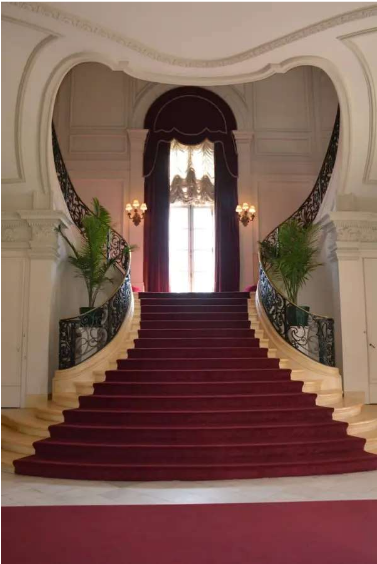
Made of Caen limestone, a cream-colored stone quarried near Caen, France, Rosecliff's signature heart-shaped staircase is most likely modeled after a similarly designed staircase in Nancy, France. The lush red velvet drapes and red carpet dramatize the heart-
